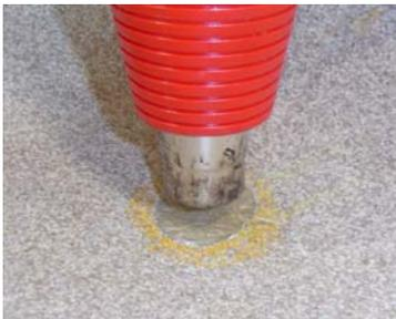
**Dry out the fiberglass with heat gun.**
