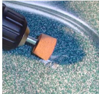
Prepare the damaged area by cutting and grinding.
