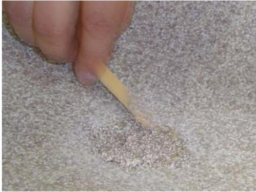
**Application – There must be an excess layer of cured repair mix, which will be sanded away.**
