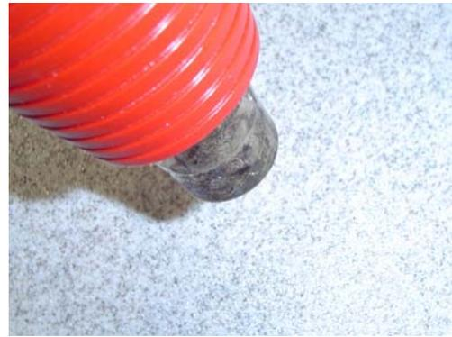
**Proper Drying Technique – Use gentle, continuous, circular heat around the edges of the applied texture.**
